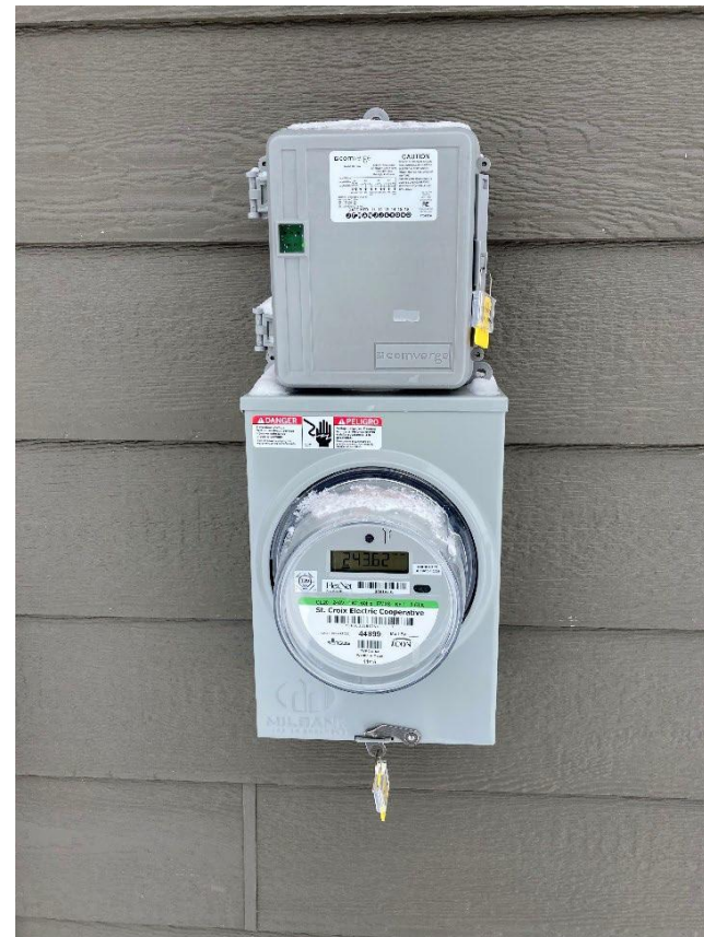
Example of off-peak installation
