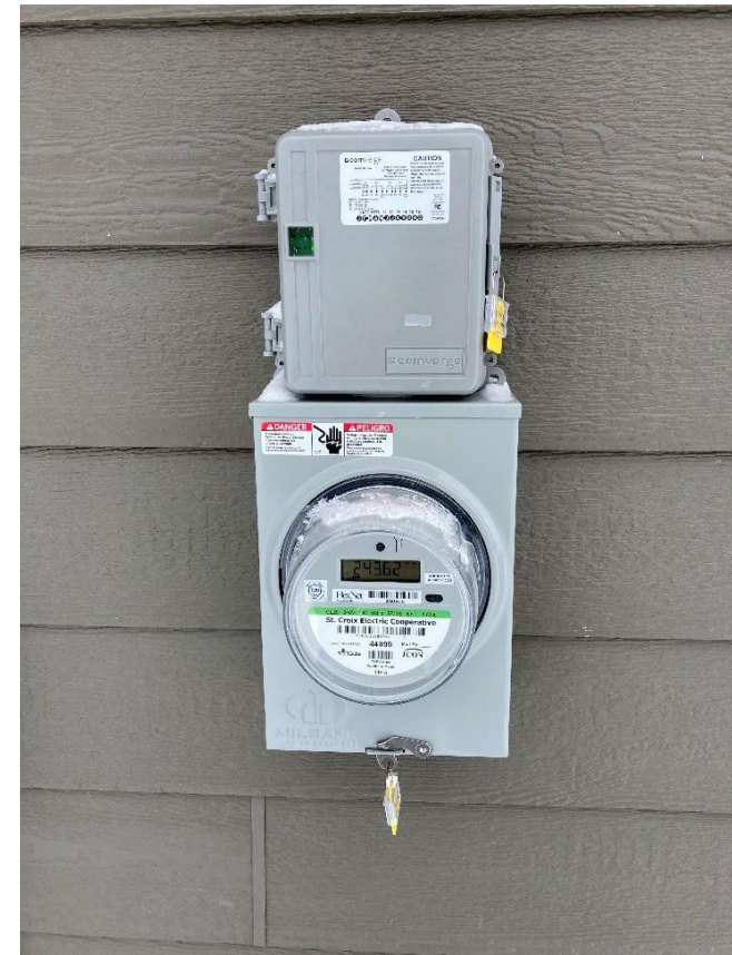
Example of off-peak installation
